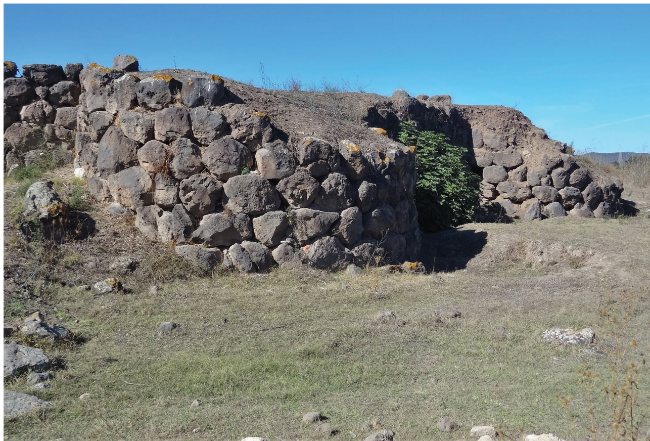
Fig. 2.7. Towers in the curtain wall of Nuraghe S'Uraki (San Vero Milis).
