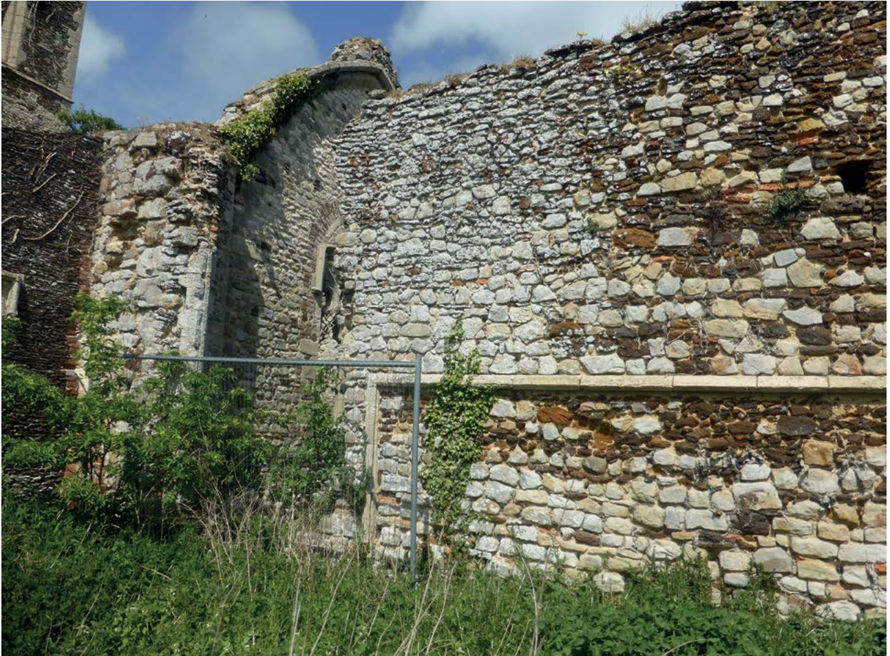
1.31. Babingley north wall interior of chancel with squared blocks of grey quartzite.
