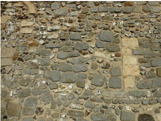
1.32. Brancaster chancel south wall with squared blocks of grey quartzite.
