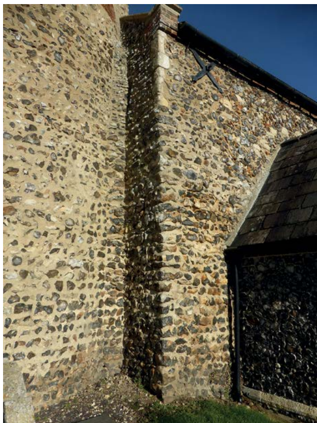
1.7. Surlingham nave south-west corner with squared flints, one piece of conglomerate and limestone near the top.
