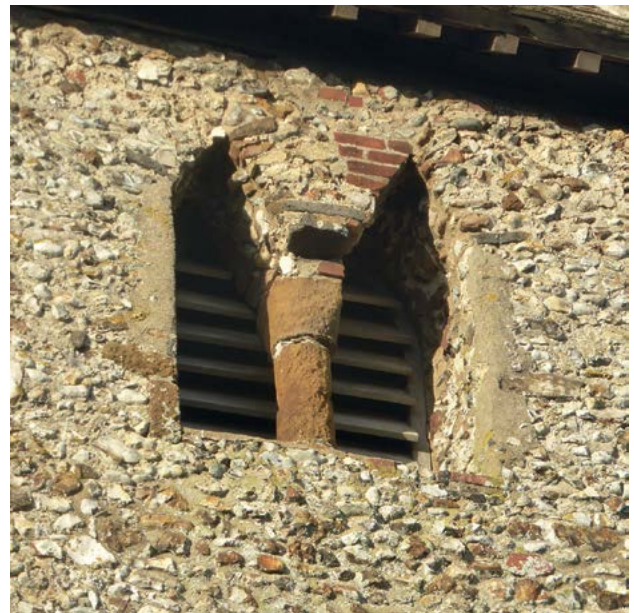
1.52. Newton by Castle Acre tower belfry window with a possible Carstone mid-wall shaft and capital. This triangular window head was rebuilt in the 1929 restoration with a mixture of conglomerate, Carstone, brick, flints and pieces of lava quernstone.
