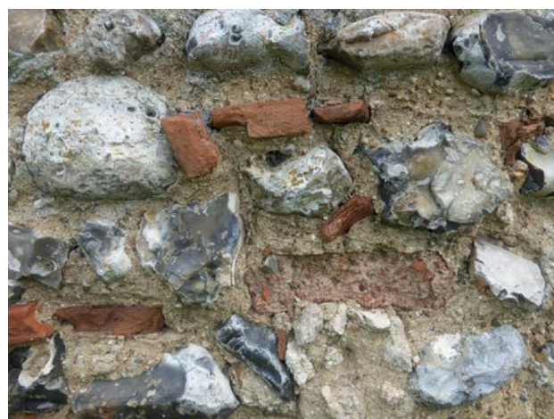
1.47. Haveringland round tower with Roman tiles and a blocks of opus signinum .
