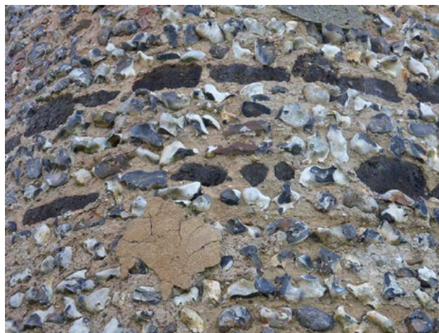
1.21. Bampton tower with a small area of lime plaster surviving in situ .
