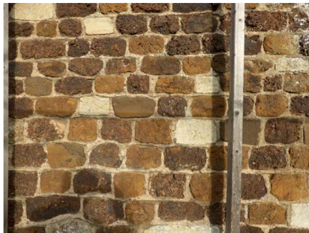
1.2. Wimbotsham south wall of the chancel which has a decorative mixture of light brown Carstone, darker brown ferruginous conglomerate and limestone.
