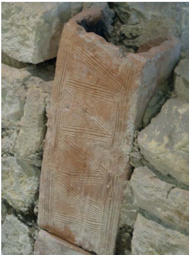
1.41. An example of a Roman flue tile in Chedworth Roman villa, Gloucestershire: not easy to recognise in churches because the scratched surface would not be exposed, although a few examples were found in the North Elmham tile collection.
