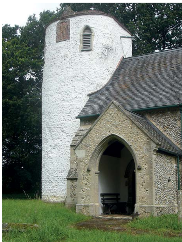
1.5. West Lexham tower after restoration with the chalk protected by multiple layers of lime water.
