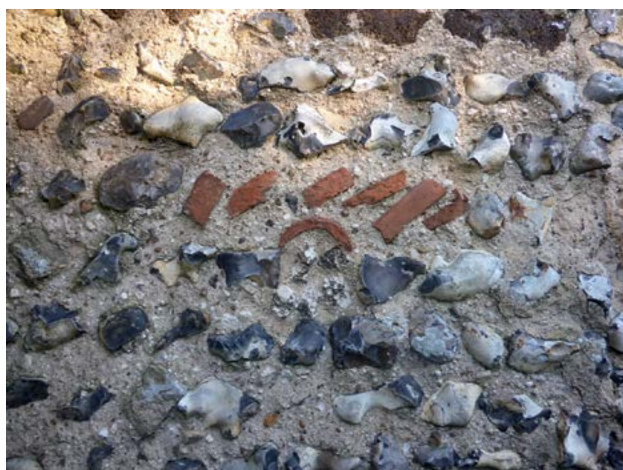
1.46. Brampton nave west wall Roman tiles including a rare example of an imbrex .
