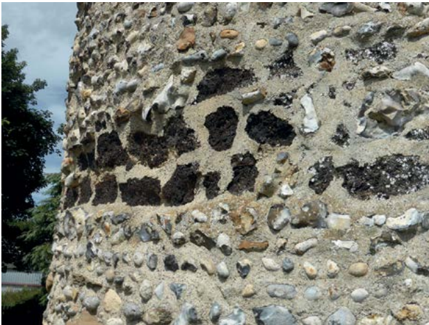
1.13. Mauthby round tower with layers of eroded conglomerate.
