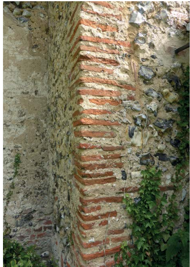
1.42. Oxnead nave south-west corner built entirely of Roman tiles
