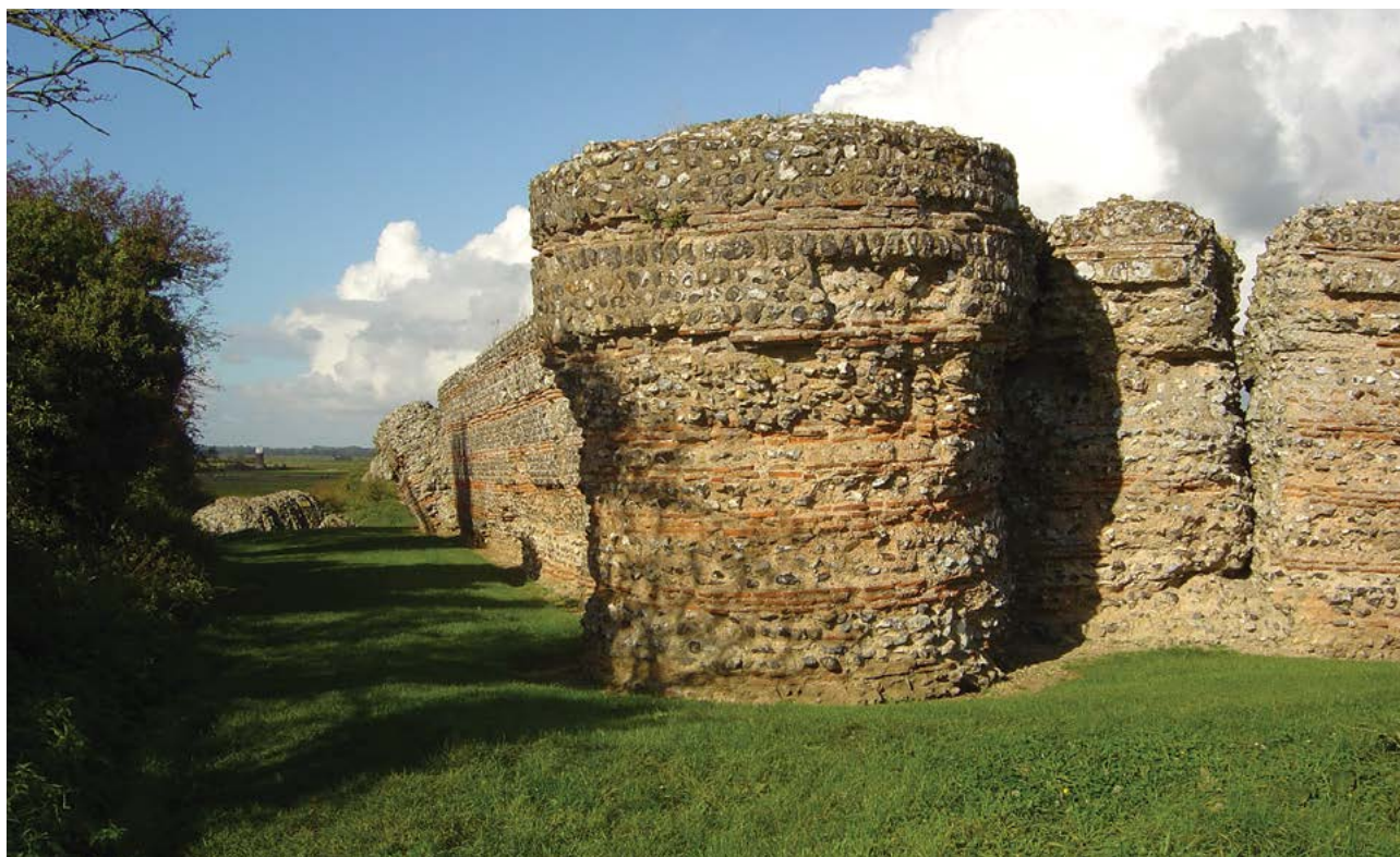
1.36. Burgh Castle Roman fort south-east bastion with layers of wall bonding tiles.
