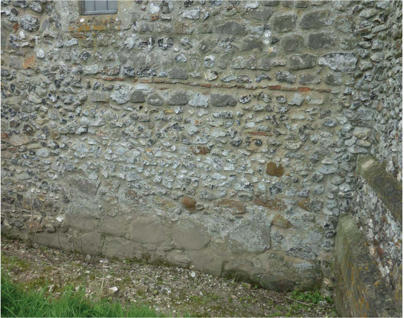
1.28. Flitcham tower north wall with blocks of grey quartzite, flints and a course of Roman tiles.
