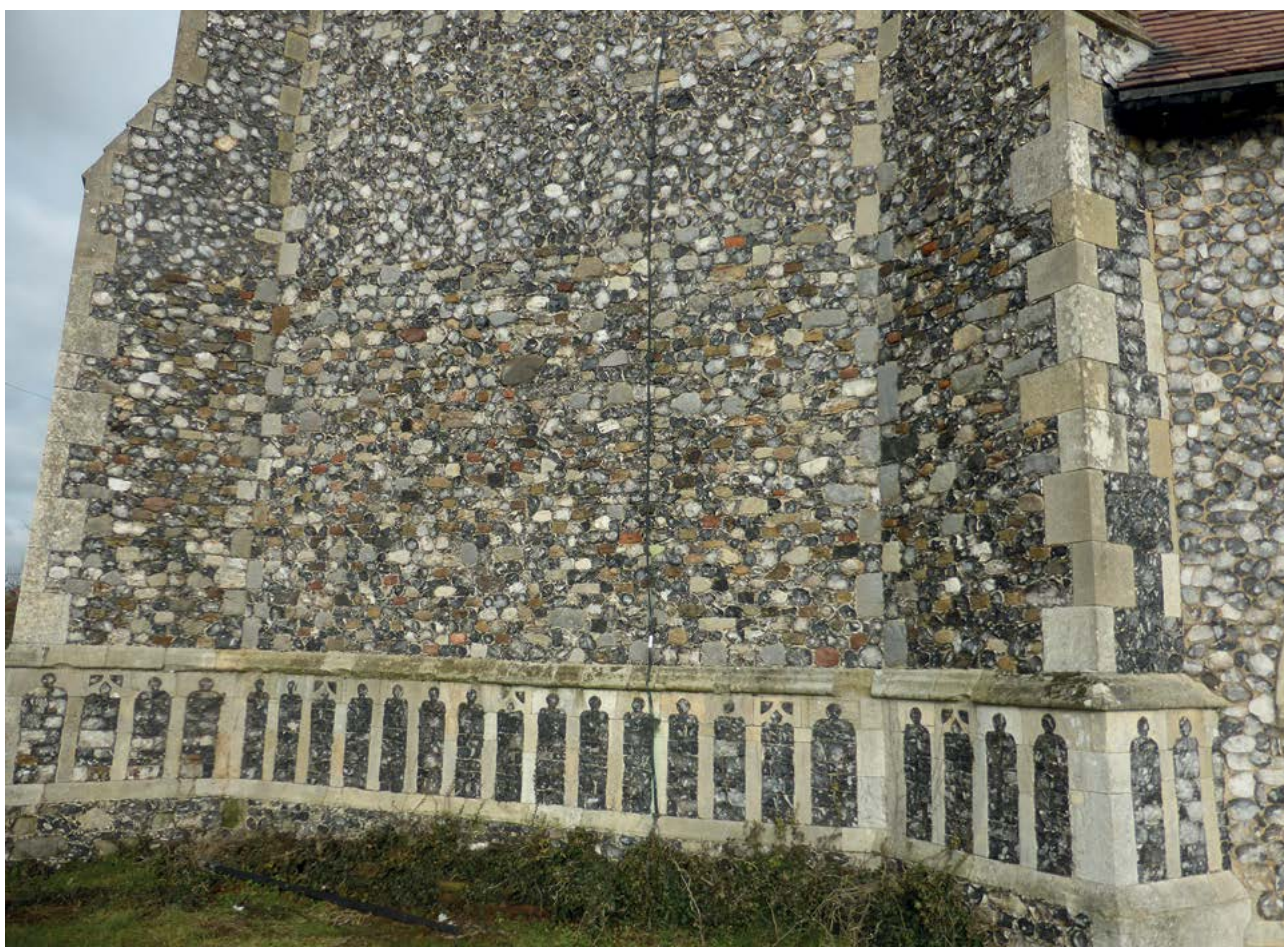
1.34. Limpenhoe tower south side with blocks of grey quartzite.
