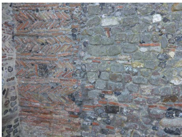
1.33. Reedham nave north wall with Roman tiles laid herringbone and grey quartzite.
