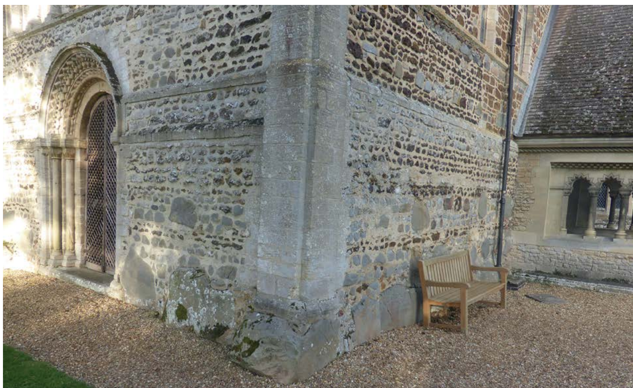
1.23. Castle Rising St Lawrence nave south-west corner with a foundation course of large blocks of grey quartzite.
