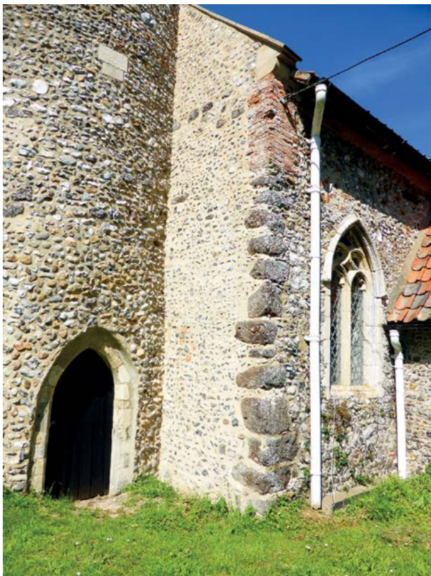
1.18. Sustead nave south-west corner with conglomerate quoins with additional tiles of uncertain date above.
