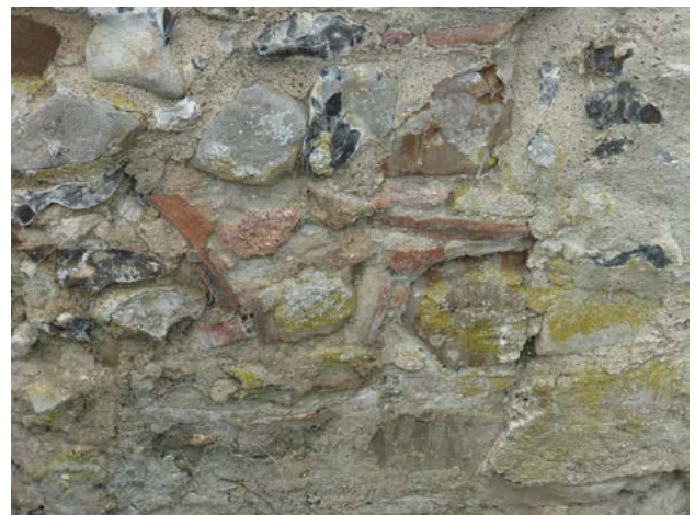
1.29. Flitcham tower east side with Roman tiles and opus signinum .
