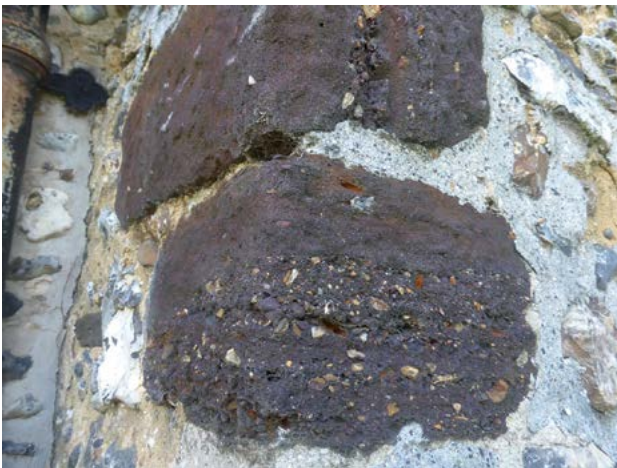
1.9. Ketteringham nave north-west corner with sandy and gravelly versions of conglomerate in the same quoins.
