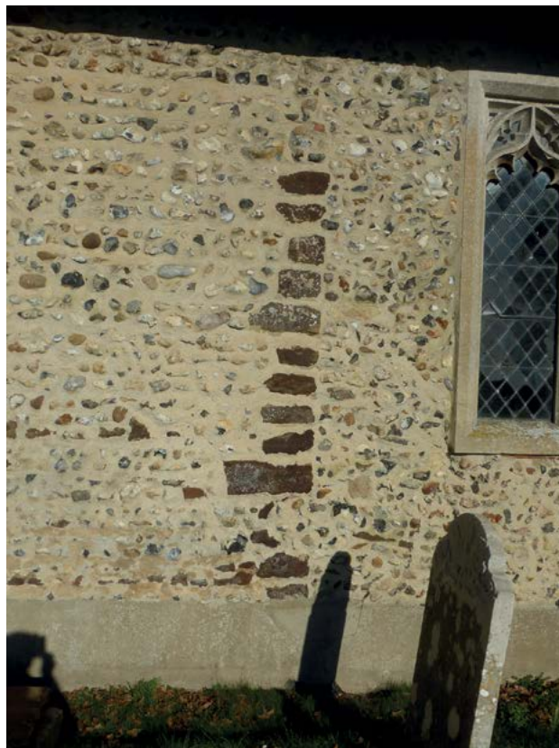
1.19. Ashby St Mary nave south-east corner showing as conglomerate quoins in the south wall where the nave and the present chancel south walls are aligned.
