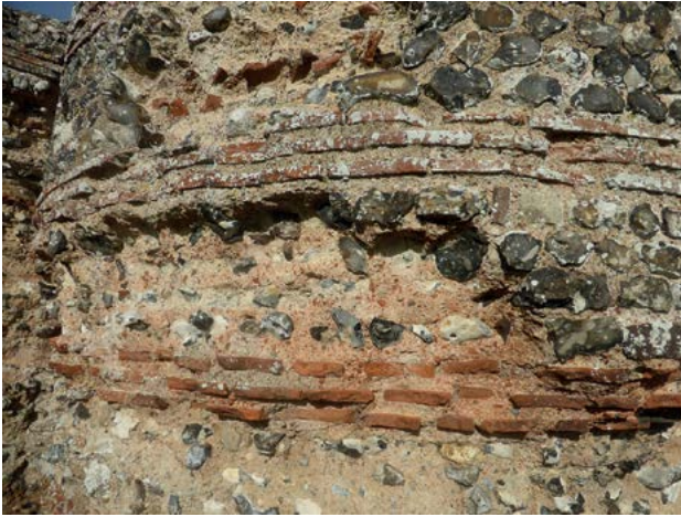
1.37. Burgh Castle Roman fort an eastern bastion with both wall bonding tiles and opus signinum .
