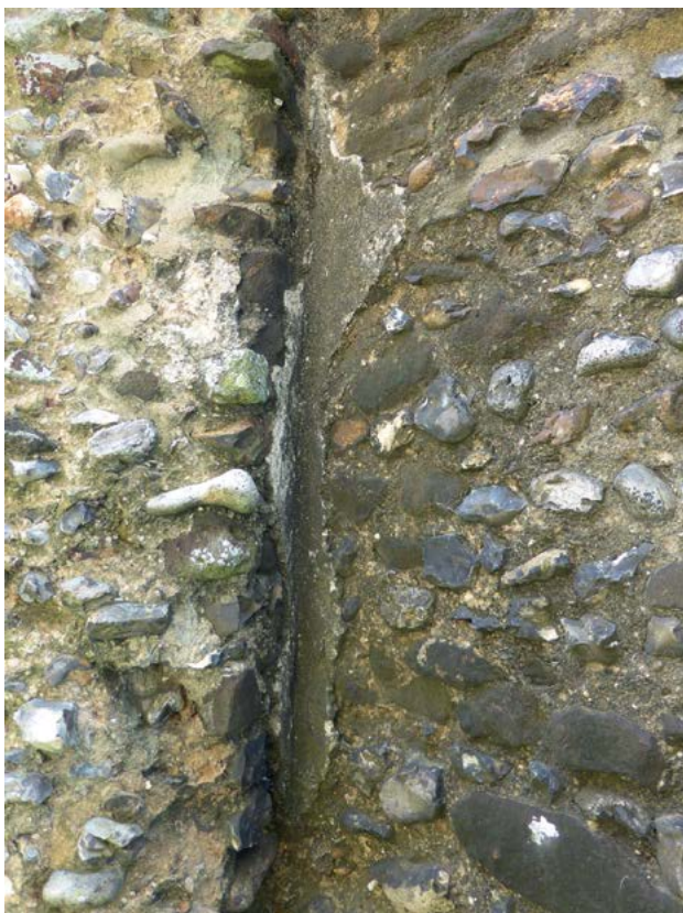
1.20. Little Snoring angle between the remaining west wall of the nave (to the left) and the tower with some surviving lime plaster.
