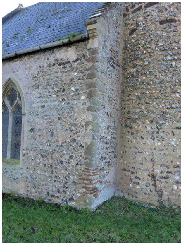
1.35. Brampton nave north-west corner with Roman tiles and grey sandstone quoins identified as a Millstone Grit.
