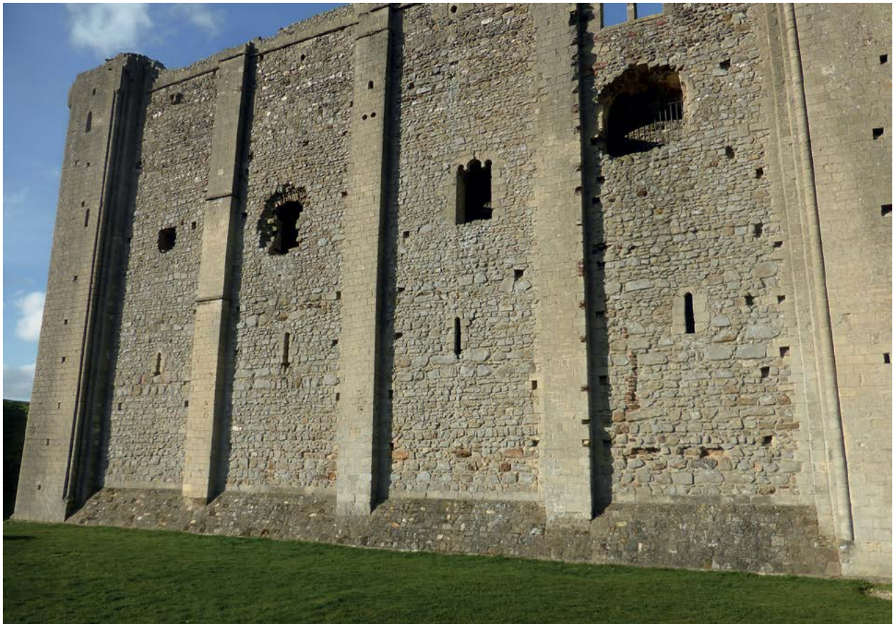
1.24. Castle Rising castle keep south side built with limestone ashlar buttresses separated by panels filled with blocks of grey quartzite of varying sizes.
