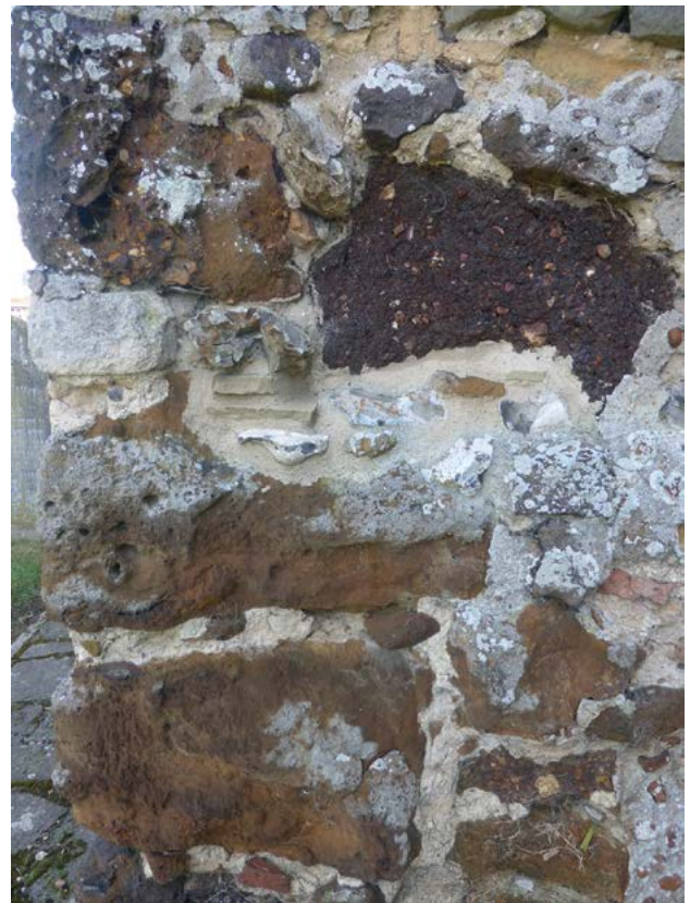
1.11. South Wootton nave north-west corner with conglomerate quoins with a mixture of light brown Carstone and a piece of darker conglomerate containing some fossil molluscs.
