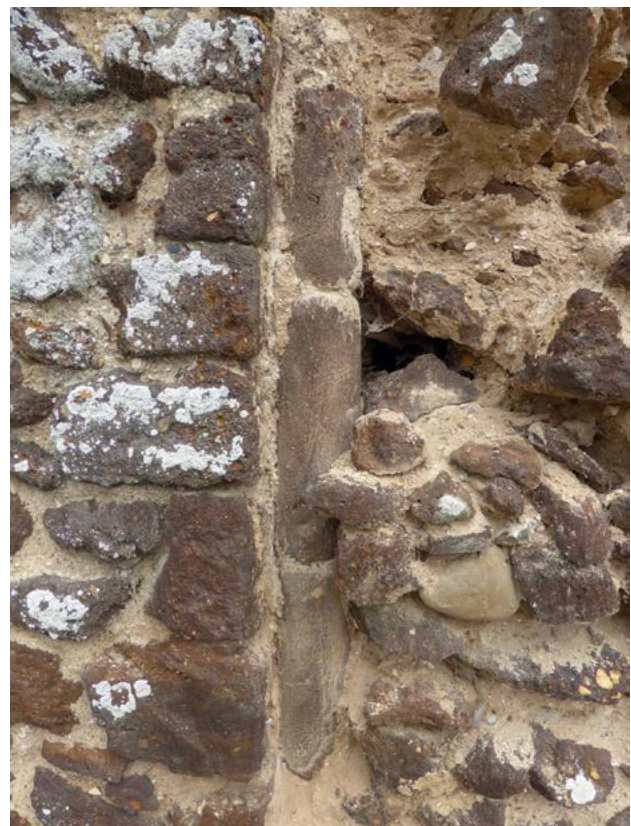
1.15. Burgh Parva nave blocked south doorway with conglomerate jambs and nook shaft.
