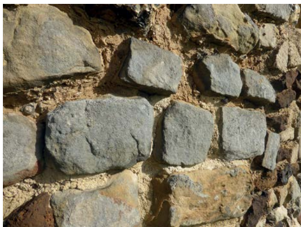
1.26. Appleton tower with grey quartzite blocks from Denbeck Roman villa nearby.
