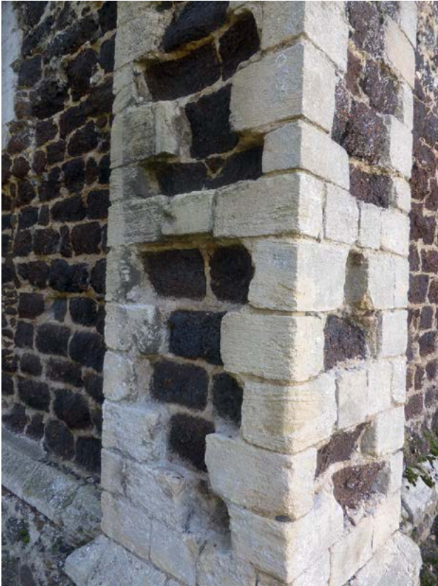
1.12. Ryston tower south-west buttress with limestone ashlar and heavily eroded conglomerate.
