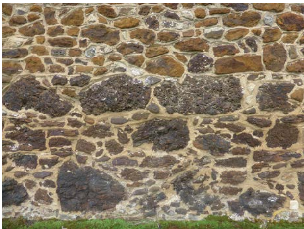
1.1. Bexwell close-up of the stonework in the east wall of the chancel wall which has a mixture of light brown Carstone and larger blocks of darker ferruginous conglomerate.
