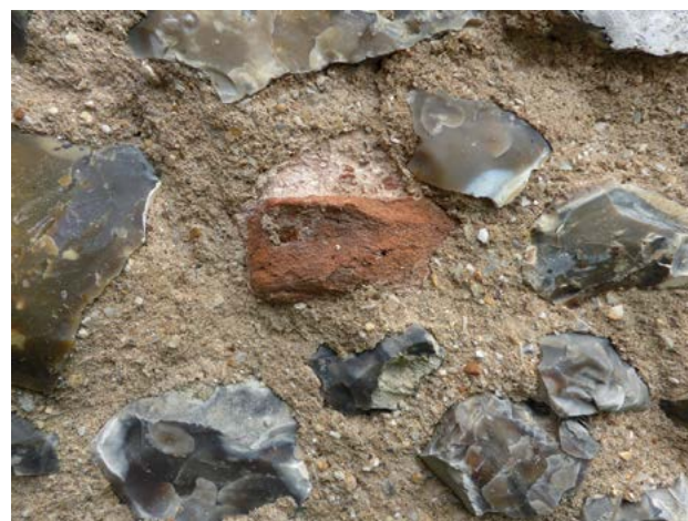
1.48. Sparham south aisle Roman tiles with opus signinum stuck to it.
