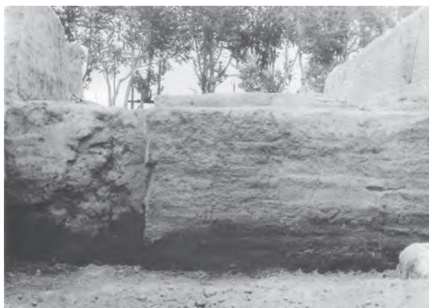
Figure 1.2. Top: the extant *hangtu* walls found at Zhengzhou Erligang. Bottom: layers of earth were pounded hard piled up. Erligang period. After Zhengzhou Shangchang 2001, pl. 7 and 39.
